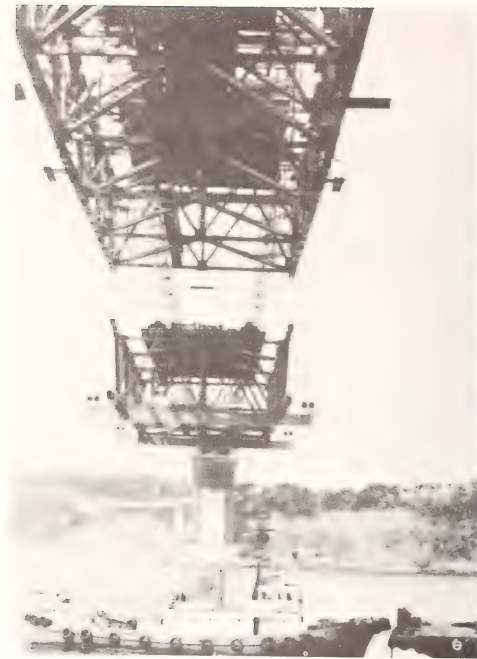
Photo-1 Erection of suspended structure
